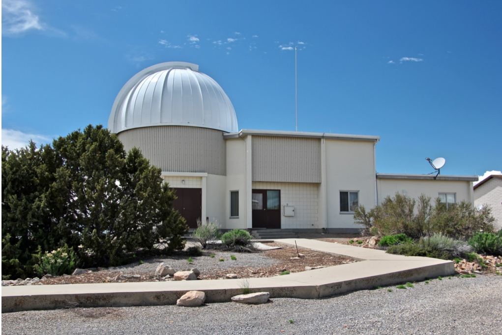
Figure 2. The main building at the BYU West Mountain Observatory looking toward the west.
